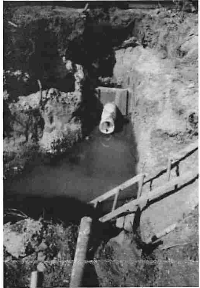
The first stage to get Hangar 604's door drains working again.
